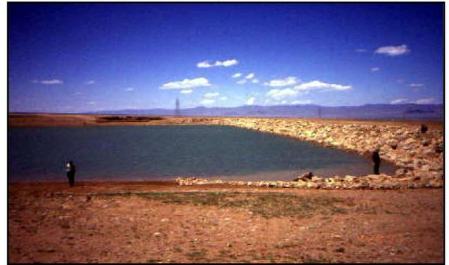
**Figure 3. Earth embankment to retain rainwater for groundwater recharge in Iran**
