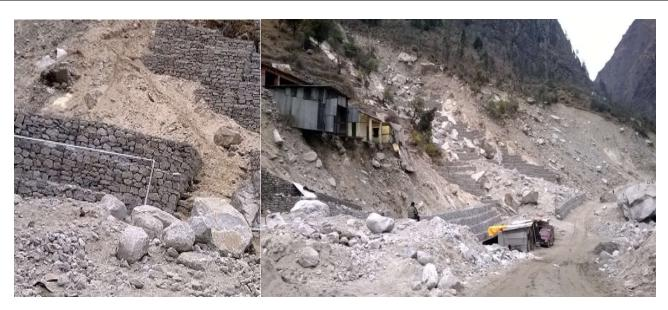
Plate 13. Inappropriate construction of retaining walls on Badrinath road near Lambagad GP
