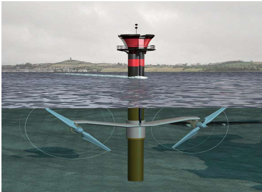
Figure 2. A Ocean turbine with protruding tower and rotating blades (Jones, 2011)
