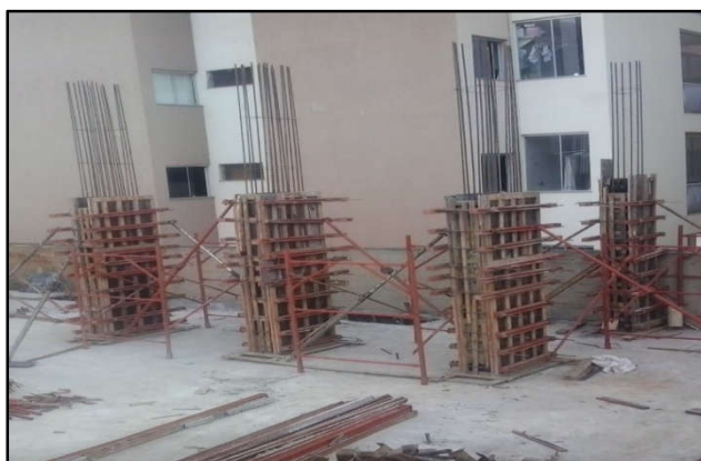
Figure 1. Mounting of the pillars rising from the foundation in the basement of the building
