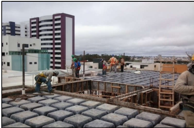
Figure 6. Positioning of the Positive Frame on the slabs of the slabs
