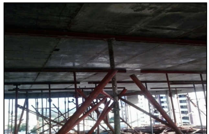
Figure 5. Shoring of slabs for placement of cuvettes
