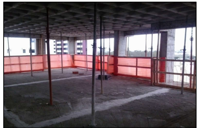
Figure 9. Ribbed slab after removal of forms
