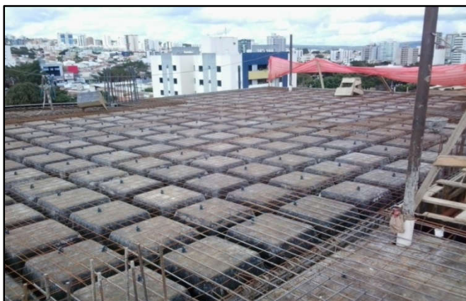
Figure 7. Positioning of the positive reinforcement in the two directions of the slab
