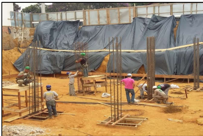
Figure 1. Mounting of the pillars rising from the foundation in the basement of the building
