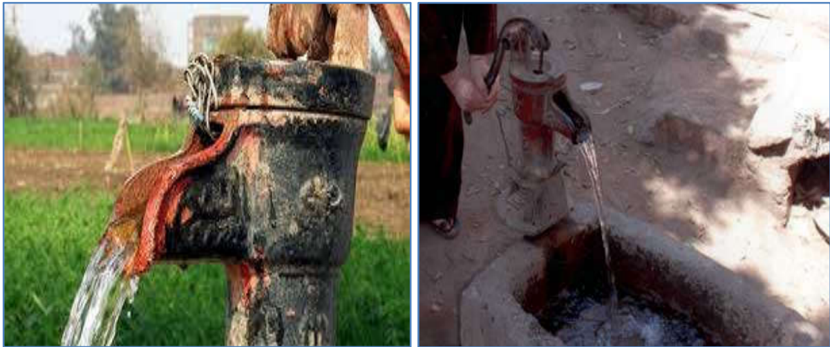
Fig. 5. Shallow water pump found in every home in rural area in Egypt (personal photos by Author)
