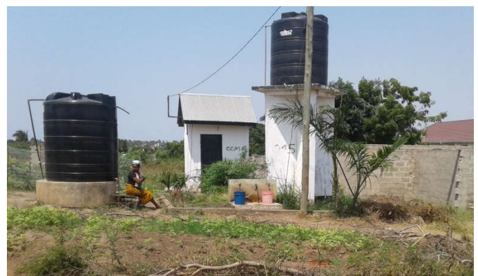
Plate 2. A water supply point under the community-based scheme at Muungano
