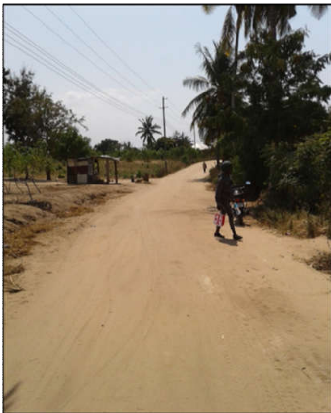
Plate 1. Road without storm water drainage system at Muungano settlement
