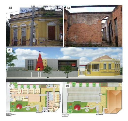
Figure 1. Casa Amarela (Yellow House) — UMEI Timbiras. View of the facade from Álvares Cabral avenue (a) Facade (b) Internal view (c) Design project of the recovery of the façade (d) Design Project of the 1st floor of the building and (e) Design Project of the 2nd floor of the building. Source: Rede Cidade (2008)
