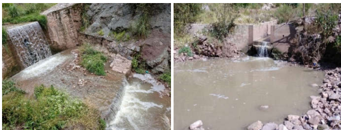
Figure 10. The Saphy River in the last section receives wastewater and has waterfall aerators that re-oxygenate the water
